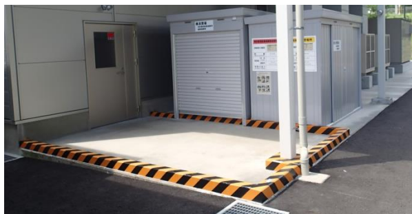
Oil retaining wall around liquid waste storage
